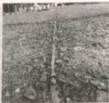
Photo 3. FOD Trapped Inside Joints
