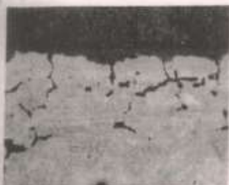
Photo 2. Damaged Edges and Sealant of Joints
