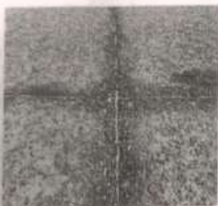
Photo 2. Damaged Edges and Sealant of Joints
