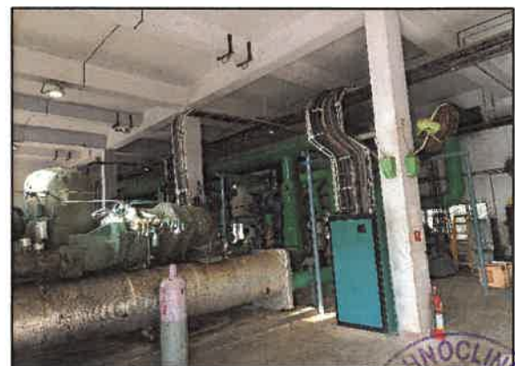
PH 02 - Internal View
