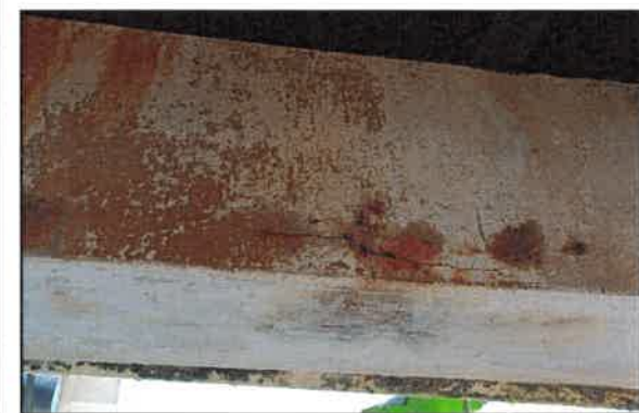
PH 06 - Severe cracks in RC members
