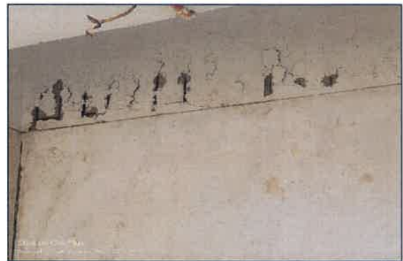
PH 08 - Cracks & exposure of corroded rebars in internal side
