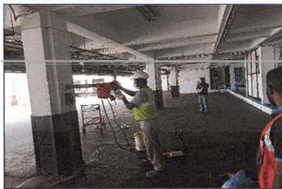
Extraction of Concrete Core Samples is in Progress
