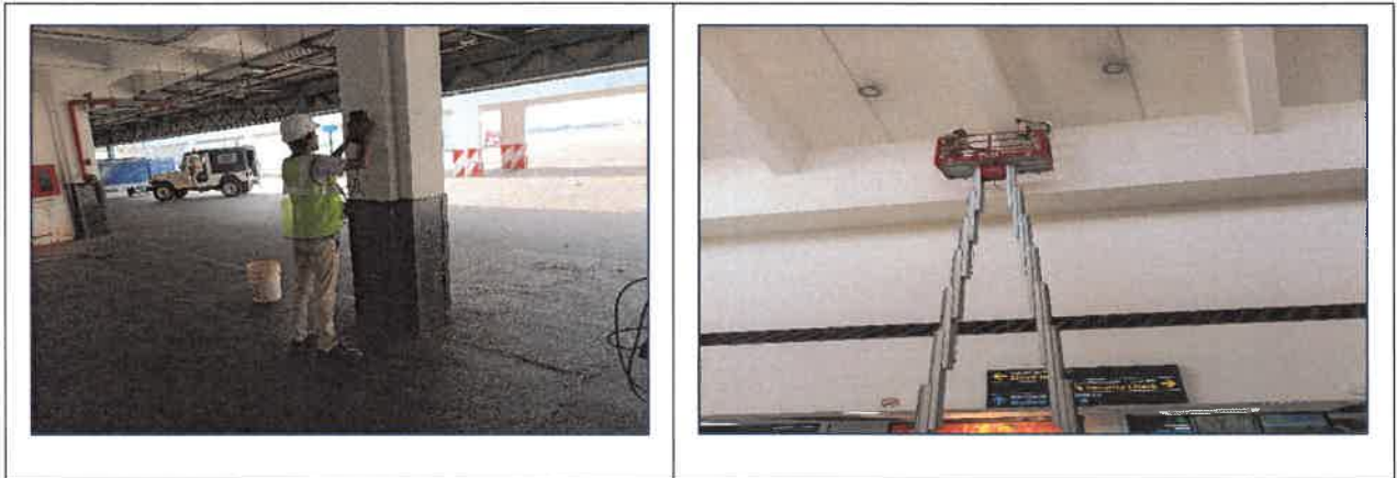
Cover Meter Test is in Progress
