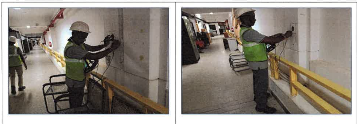
Half-Cell Potentail Measurement Test is in Progress
